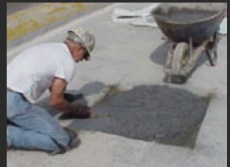
Placing SW-81 Repair Mortar
