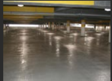
Finishing Installed Strongcote Coating
