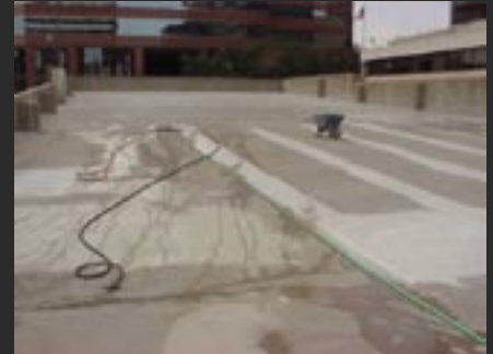
Strongcote During Installation
