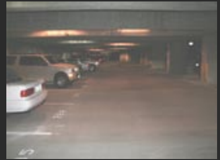
Parking Deck After Strongcote Installation
