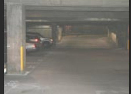
Parking Deck After Strongcote Installation
