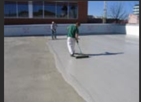
Installing Strongcote Membrane
