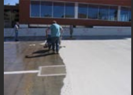
Installing Strongcote Membrane
