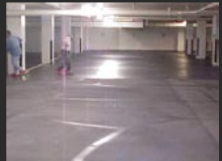
Installing SC-113 System
