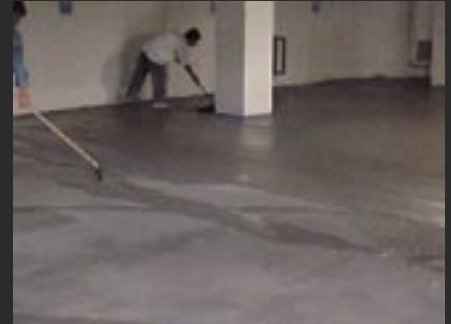
Installing SC-113 System
