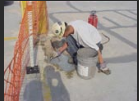
Extensive Concrete Repair Using SW-81
