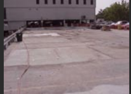
Extensive Concrete Repair Using SW-81
