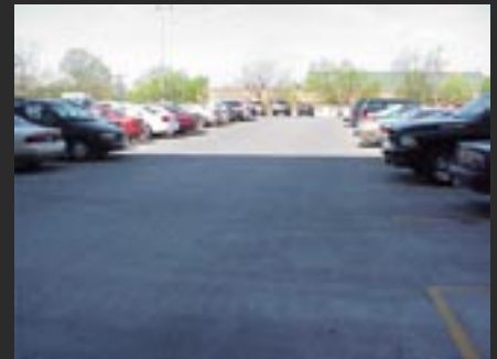
Finished Deck Coating
