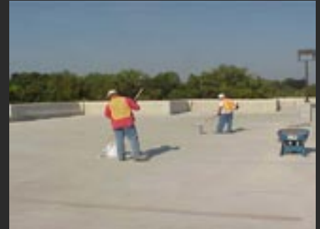
Detailing Cracks Using EM-100N
