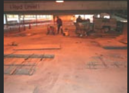
Extensive Concrete Repair Using SW-81
