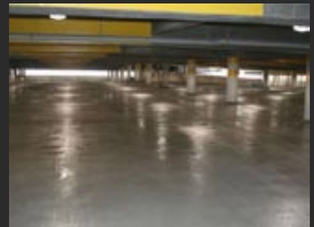
Finished Deck Coating
