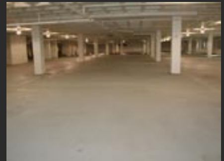
Finished SC-113 System
