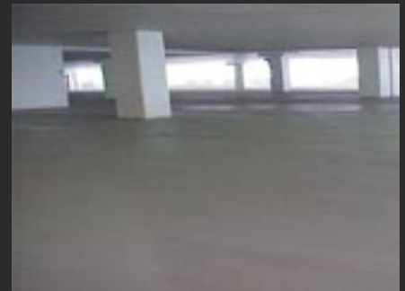
Finished SC-113 System
