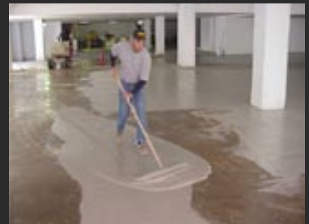
Installing Membrane
