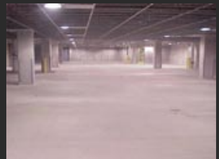
Finished Traffic Coating System
