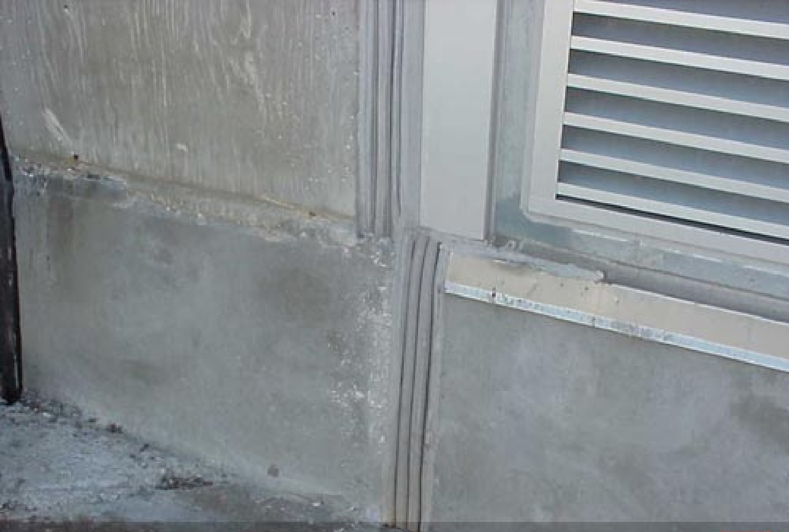
Seismic Color Seal At Concrete Joint
