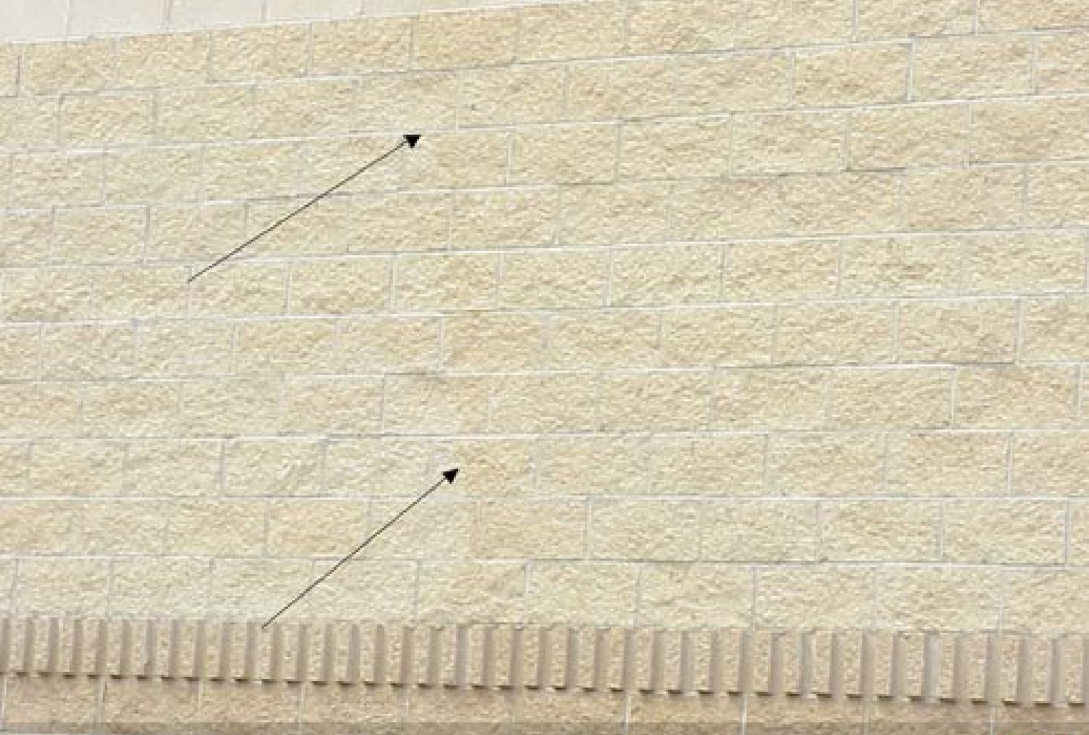
Aquafrete Immediately After Placement, Before Curing
