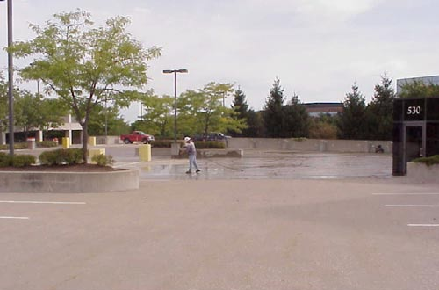
Power Washing Deck Before Treatment
