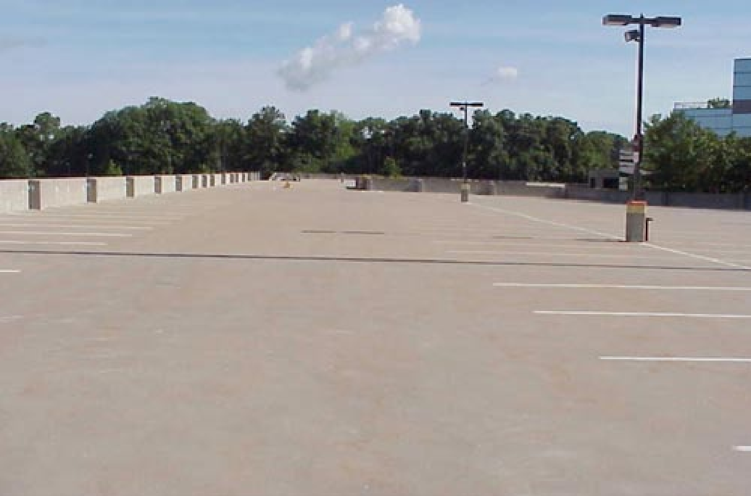
Deck Area Before Sealer Treatment
