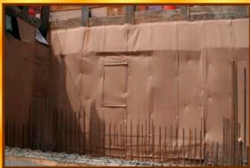
Ultraseal SP Attached to Shotcrete Retention
