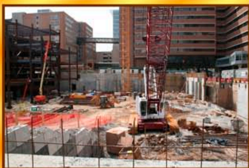
Overview of Job Site
