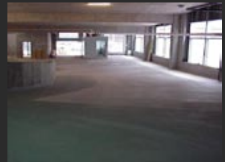
Main Ramp After Preparation And Coating
