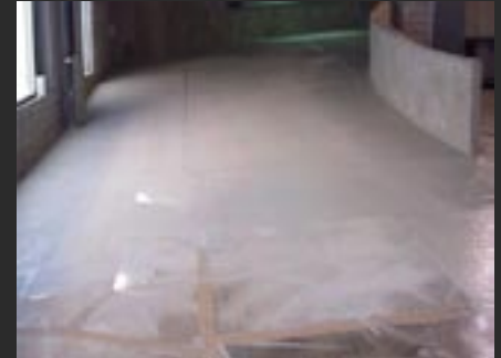
Main Ramp After Preparation And Coating
