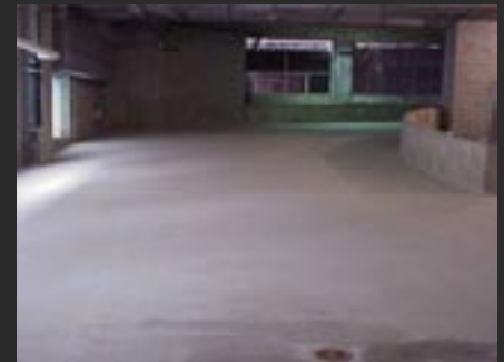
Finished Traffic Coating
