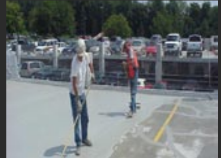
Installing Coating System
