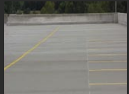
Finished SC-113 System
