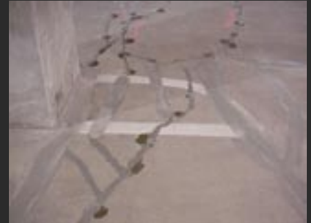
Crack Treatment Using EM-100N
